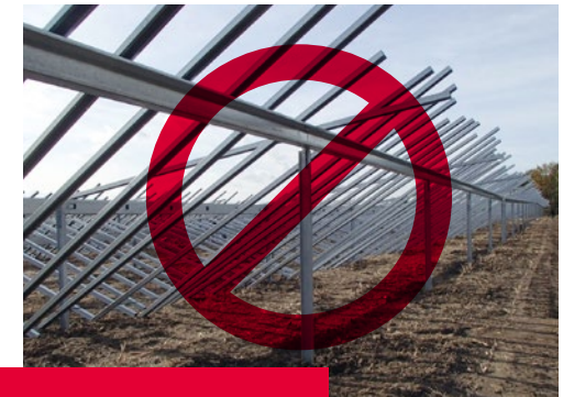
No complex substructure
